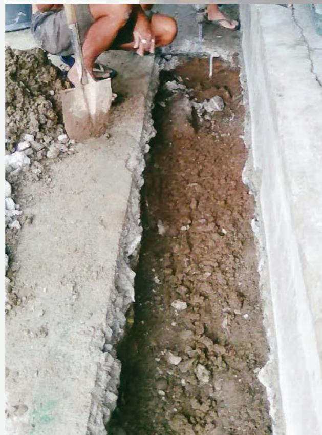
The trench drainage system of the second court worked so well during the rainy season that we decided to replicate the system in Court 1, which was experiencing some drainage problems during heavy rains. Thus, last July 2018, a trench drainage system was also built around Court 1. The new system made it easier and safer for the players to play because the water now flowed freely out of the court, no longer flooding the inside.
